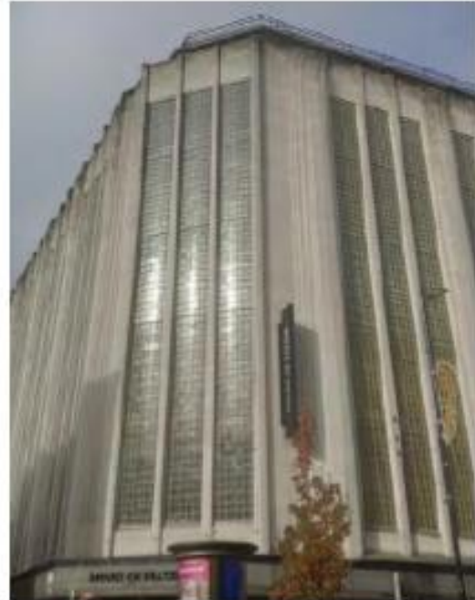
Figure 29 – An external view of the glass block windows, illustrating the subtle reflection of light. (Source: SLHA)
