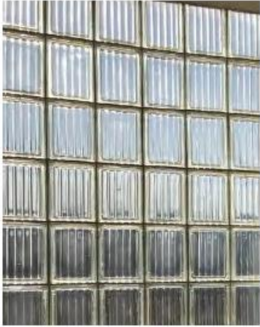
Figure 28– An internal view of the glass blocks from a shop floor. (Source: SLHA)
